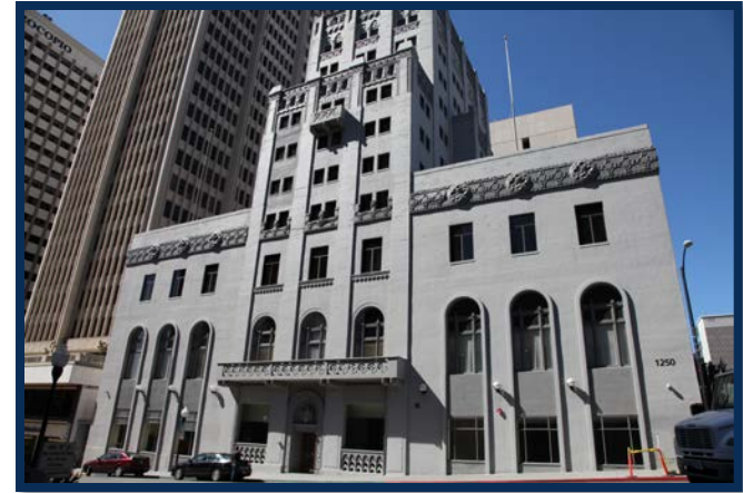
Connections Housing SDHC Partnership Program
